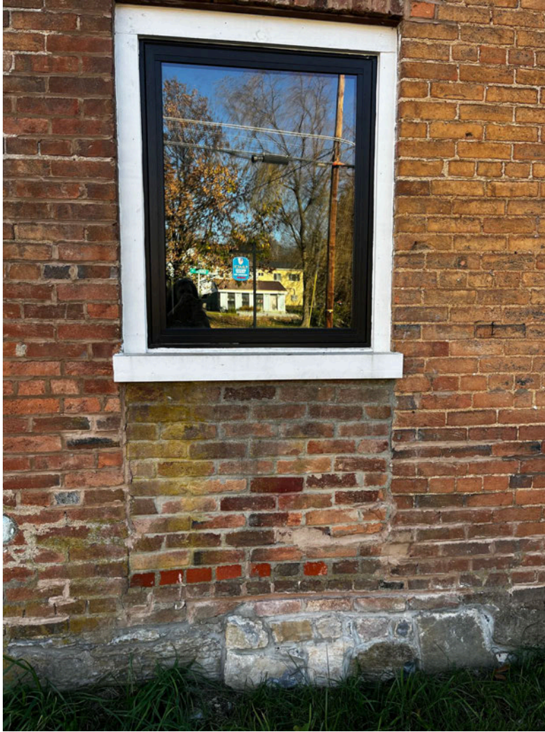
This is an example of mismatched bricks after the structure was hit by a vehicle. (Middleway, WV)
